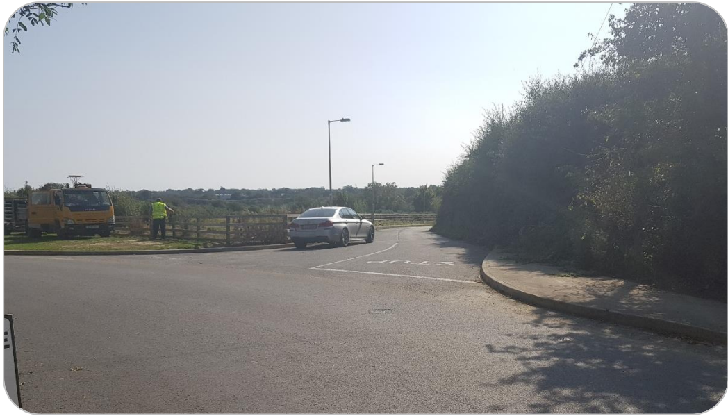
Figure 13 – Proposed primary access location on Clonattin Village (view to south) (source: CS Consulting)
